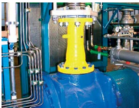
Gas Turbine Installation
